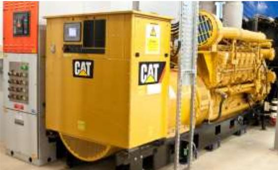
facility has been designed from the ground up with 2N resilience. This is delivered via 2 diverse power feeds from the mains supply running in parallel into the data hall and backed up with separate generators
