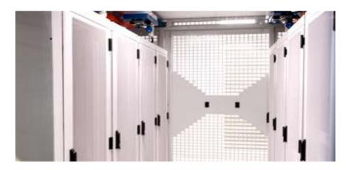
If you are completely new to talking in terms of racks, a standard rack is often referred to as a 42U-sized rack. U describes the amount (unit) of vertical space (1.75 vertical inches) that rack-mountable gear takes up in a standard 19-inch rack.
